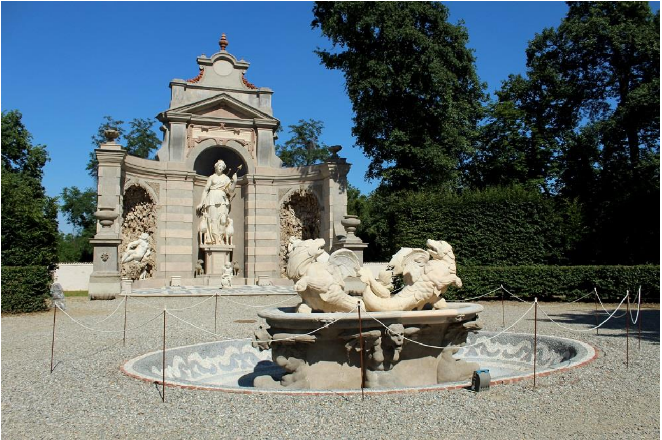
Diana's theater after the restoration completed in spring 2020
